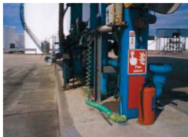
Figure 2. Typical bottom loading stand with provision for making earth connection to a tanker truck
